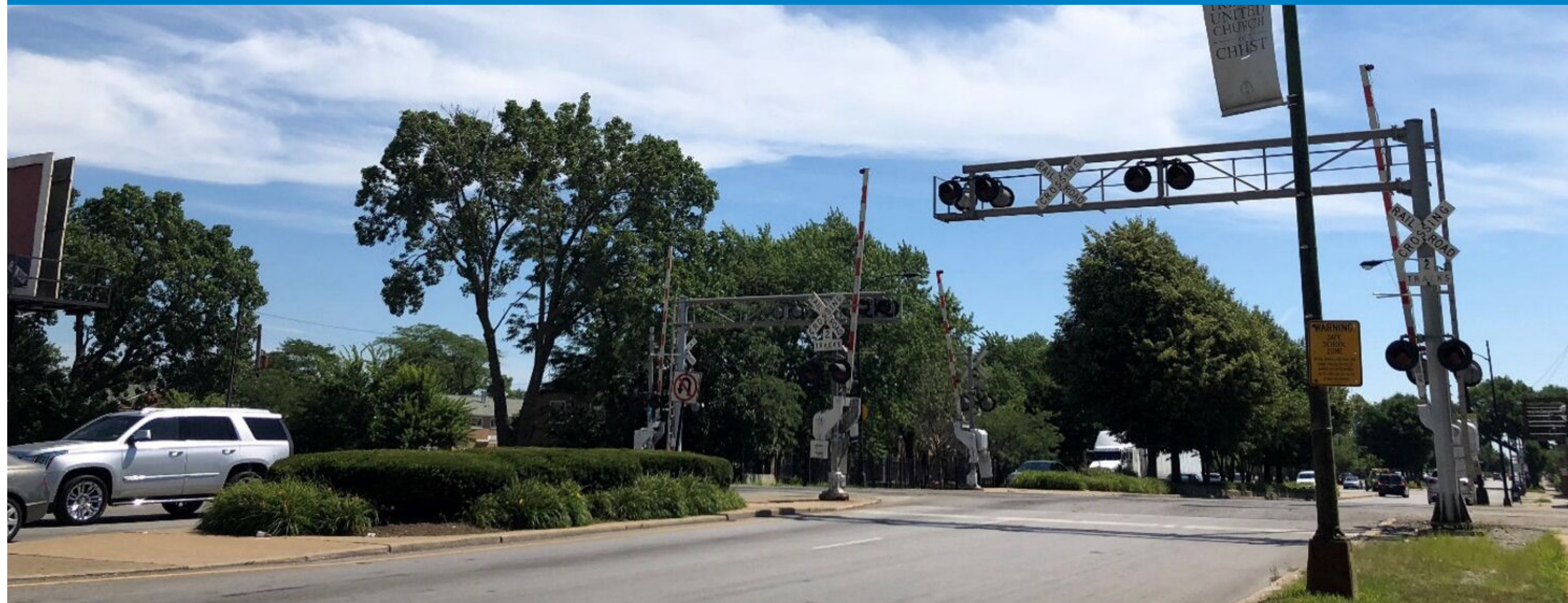
No improvement to the UPRR at grade crossing at 95th Street.
